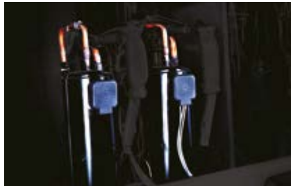
Multiple large-capacity all inverter compressors (from 14 HP).
