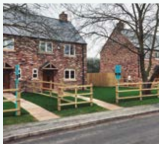
Aquarea Heat Pumps provide heating and hot water for new rural housing development, UK. Aquarea
