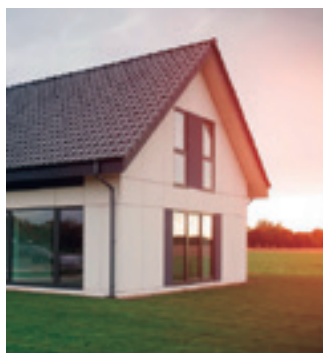
Passive house in Tychowo near Stargard Szczecinski, Poland. Aquarea
