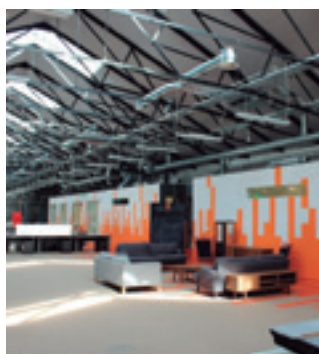
Zalando's solution for its warehouse office conversion at Grand Canal Quay, Dublin. ECOi
