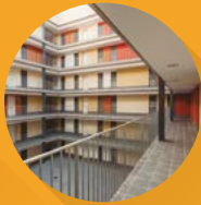
New condominium. Bergås Terrasse complex. Drammen, Norway. Aquarea
