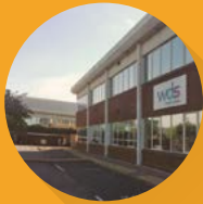
Call centre retrofit. Woodhouse Environmental Services Ltd. Bourne, UK. VRV
